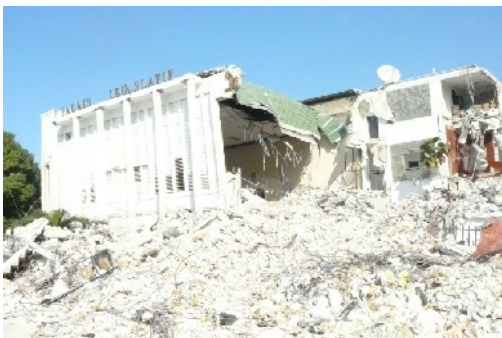
Haitian National Assembly Building
